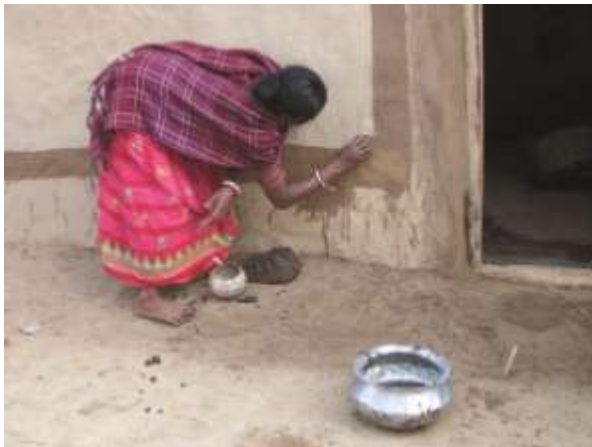
Figure 3c. Water with soft clay from agricultural field being applied on clay-wall
