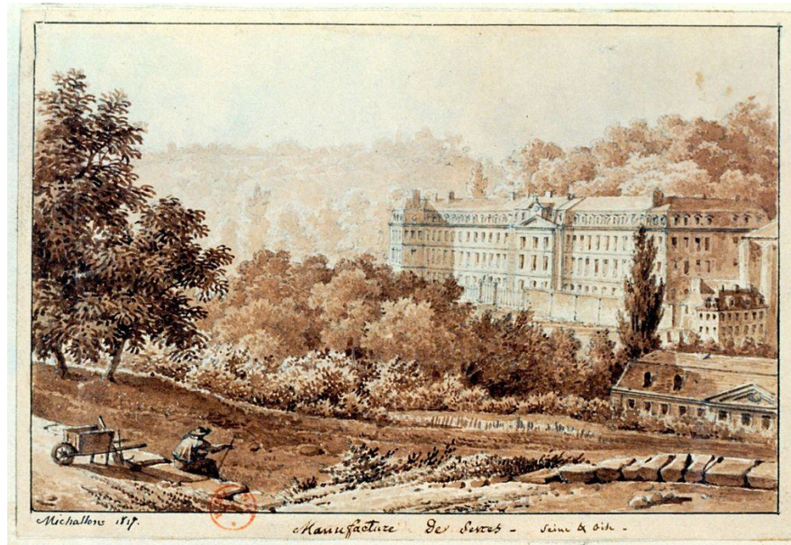
Figure 1. The Sèvres' factory in early 1800 as it was depicted by the French painter Achille Etna Michallon, (Source: Bibliothèque Nationale de France).
