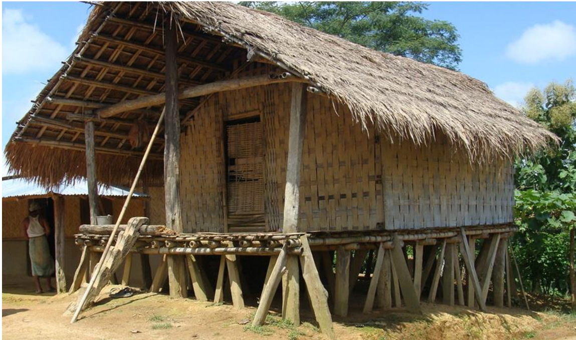
Figure 3.A Reang house or Chuklanok with thatch grass or dry bamboo leaf roof and bamboo construction.
