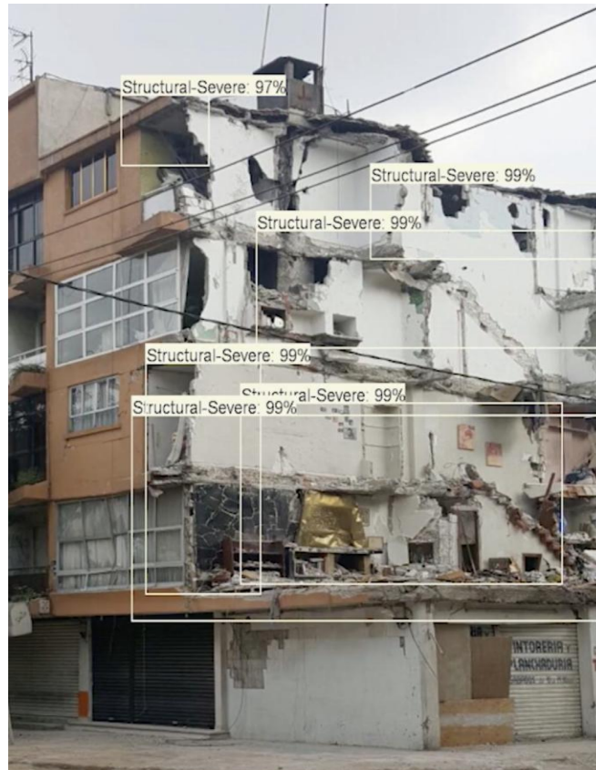
Figures 13, 14, 15: An analysis with SOM's machine learning model for structural damage (Skidmore, n.d.)
